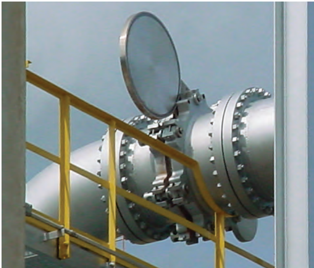
Stacey DN 850 (34") with counterweight
