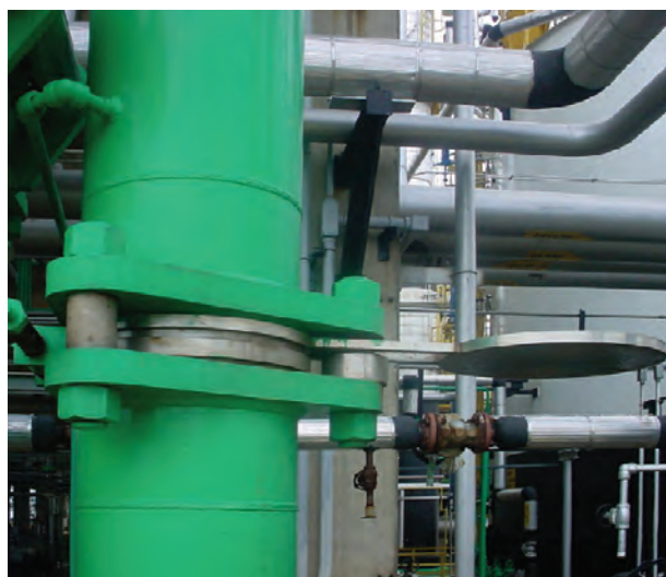
Cam-Set DN 150 (6"), ASME 150#
