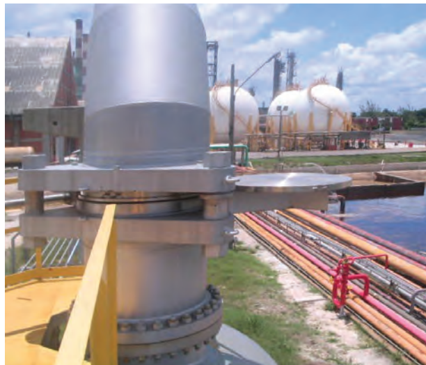
Cam-Set DN 500 (20"), ASME 150 # with spectacle plate support
