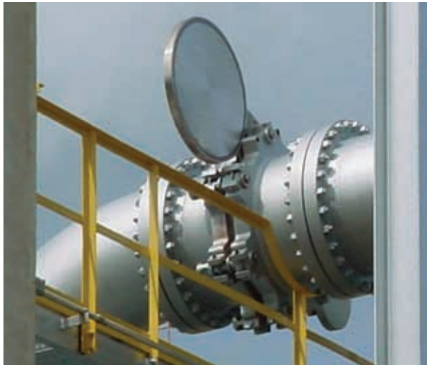
Stacey DN 850 (34") with counterweight
