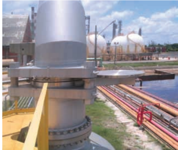
Cam-Set® DN 500 (20"), ASME 150# with spectacle plate support
