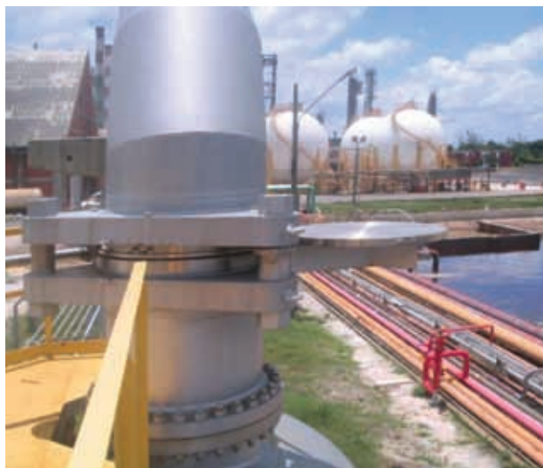
Cam-Set® DN 500 (20"), ASME 150# with spectacle plate support
