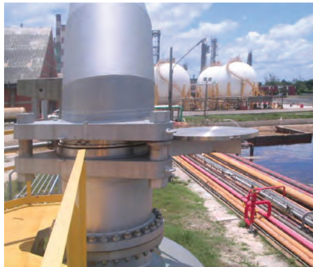
Cam-Set DN 500 (20"), ASME 150 # with spectacle plate support
