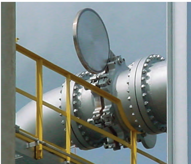
Stacey DN 850 (34") with counterweight
